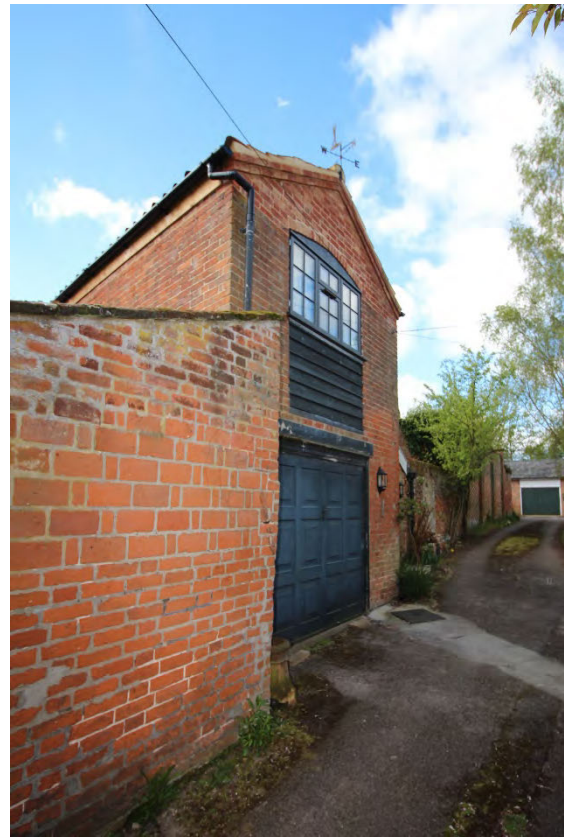
Converted Workshop to rear of Milestone House
