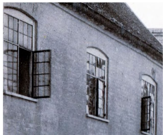
Typical Casement Windows at [redacted] now removed
