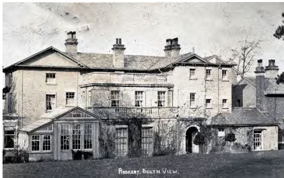
Southern façade of Rookery Park
