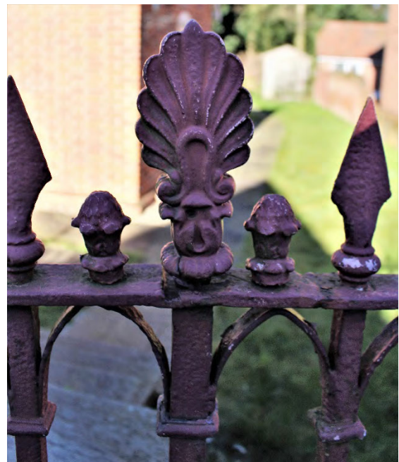
Detail of railings to Cockfield Hall's lodges
