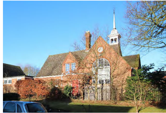
Oakwood Park façade of Yoxford School
