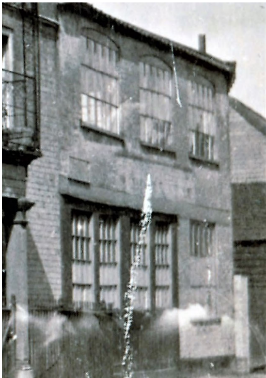
Detail of a 1918 view of Cotton's Yard
