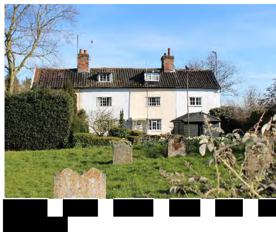
Nos.1-4 (cons), Church Lane An attractive picturesque row of four two storey cottages with attics, which are prominently located on the edge of the churchyard. Of late eighteenth
