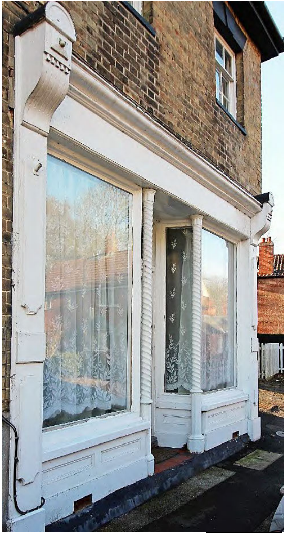
Later nineteenth century shopfront High Street
