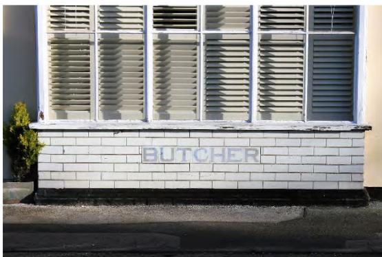
Early twentieth century shop front
