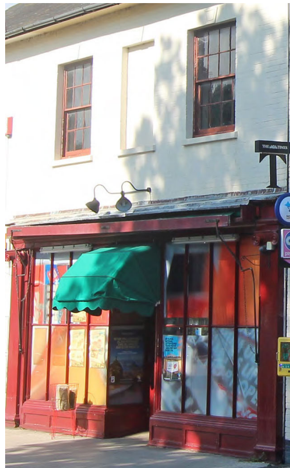
Nineteenth shopfront at
