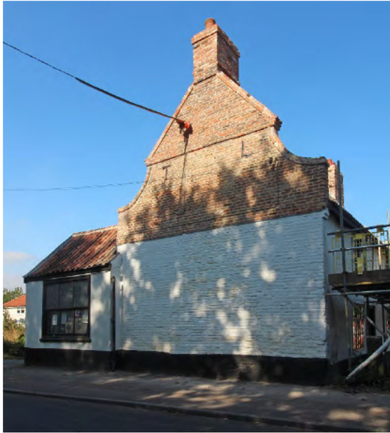
Later seventeenth century brickwork, Coal Yard House
