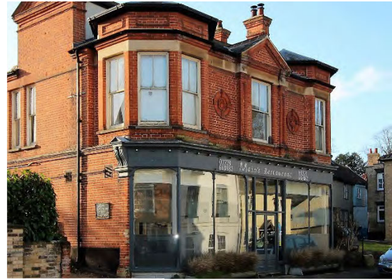
shopfront of c1902 has been adapted but remains largely intact.
